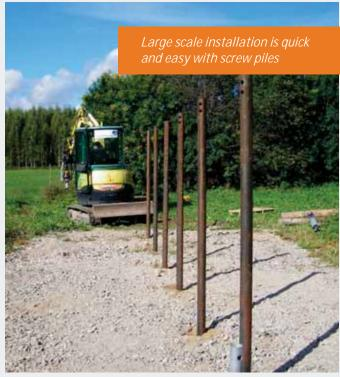
They are also environmentally friendly, as they're reusable and don't contaminate the ground or use concrete. Simply screw them in, attach the panels, and reap the benefits of clean energy.
